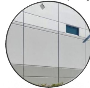
STAIN PRECAST CONCRETE (to make artificial openings)
