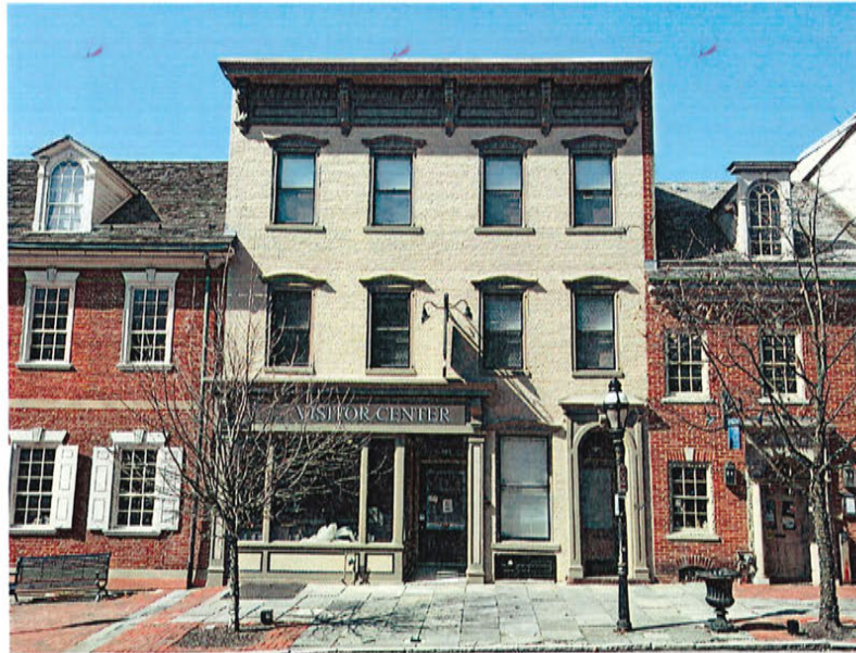
a. Schropp Schoppe and adjacent structures -- East Elevation (facing Main Street)
