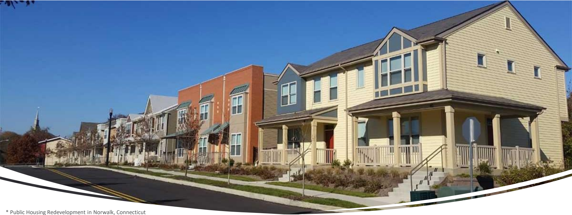
* Public Housing Redevelopment in Norwalk, Connecticut
