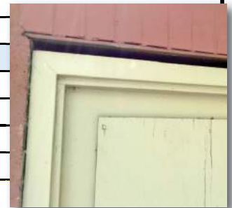
Separation of door frame from structure.
