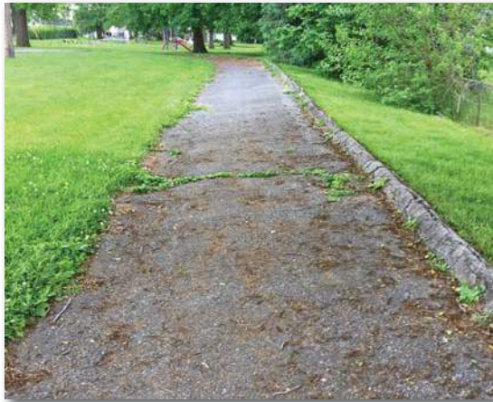
Bituminous path connecting Allwood and Grove Roads. Condition does not meet ADA criteria for smooth surface, cross slope and width.
