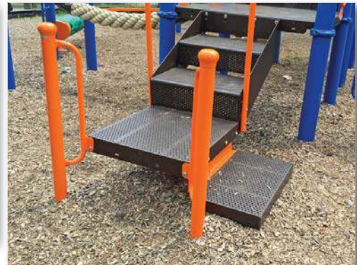
Modular play set with transfer station and appropriate mulching
