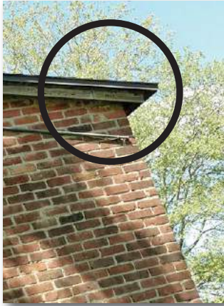
Rotting and insect damaged fascia board.
