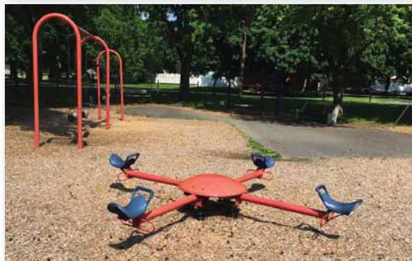
Play equipment generally does not meet current safety standards or accessibility guidelines. Inconsistent mulch depth and fall zones. Not inclusive. Bituminous areas provide limited accessibility. No sidewalks on roads surrounding this park.
