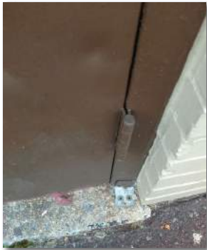
Damaged /rotting door frame
