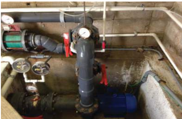
Corroded Flow Control Valve
