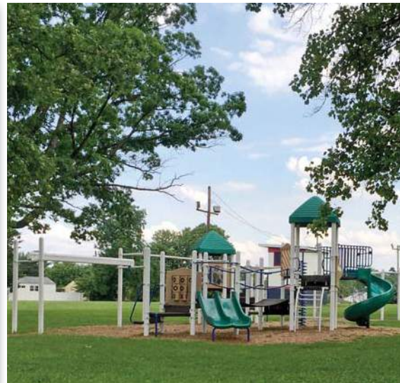
Newer playground equipment with mulch bed. Fall zones not compliant.
