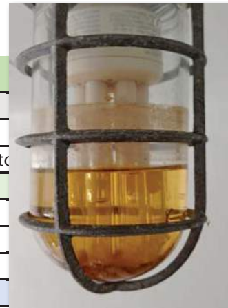
Ceiling light fixture full of water.
