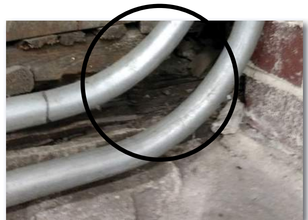
Rotted sill plate.
