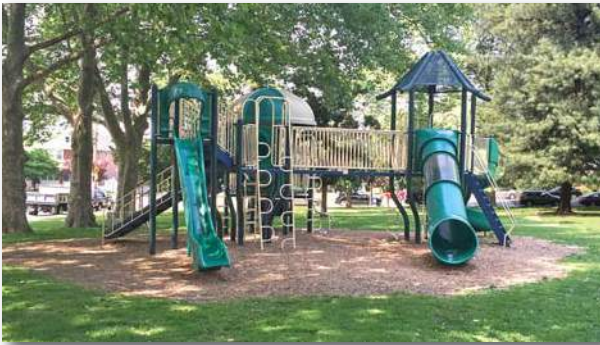
Modular Play Structure in Good Condition, Fall Zones may be inadequate
