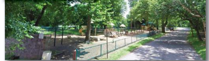
Playground - Inset shows wood members with signs of decay
