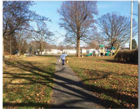
Bituminous path connecting Allwood and Grove Roads. Condition does not meet ADA criteria for smooth surface, cross slope and width.
