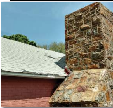
Missing/damaged shingles. Cricket and flashing show wear and damage.
