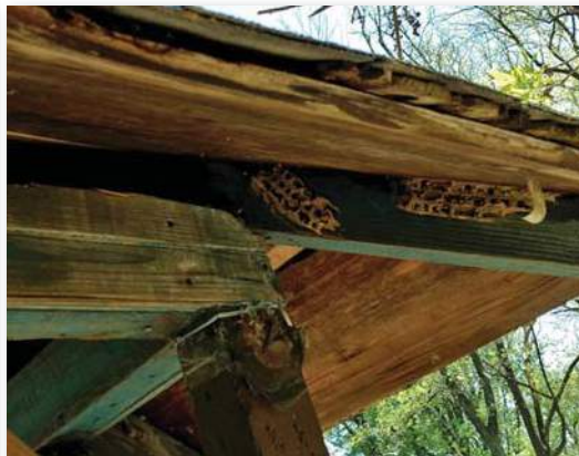
Pavilion #3: Deteriorated structural columns and roof edges.
