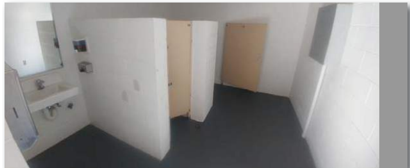
Toilet Building interior is in good condition, but do not meet current ADA criteria
