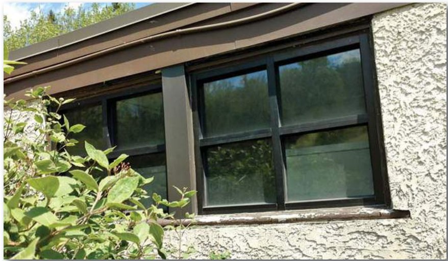
Rotting Window Sills and Warped and Damaged fascia on building exterior
