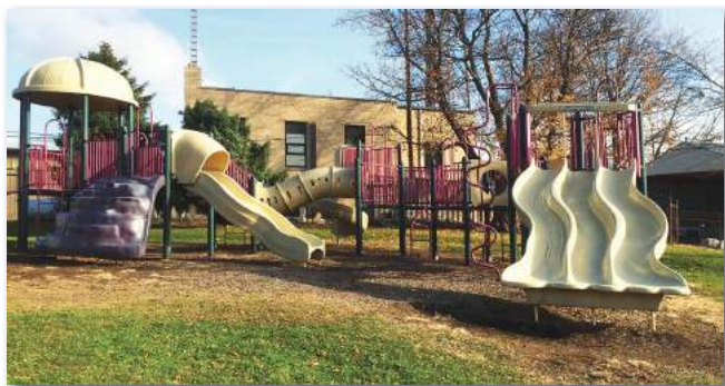
Play equipment vandalized, lacking paint, mulch & fall zone protection
