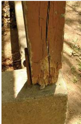
Pavilion #3: Deteriorated structural columns and roof edges.
