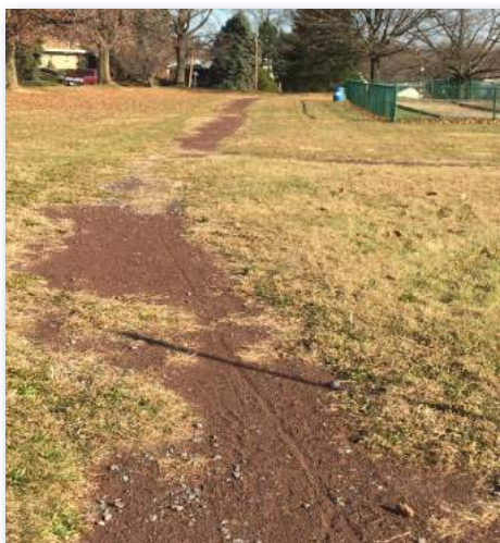
Existing Gravel Pathways becoming overgrown (typical)
