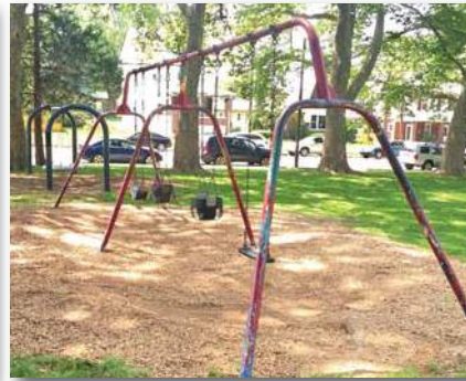
Dated Swing Frame with Peeling Paint may be Lead Hazard. Mulch pit irregular
