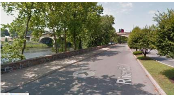
Entrance Drive to Sand Island West. Walk along WPA wall with view of the Lehigh River. Boarded areas block steep steps down to the river.
