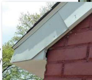
Missing/damaged shingles. Cricket and flashing show wear and damage.
