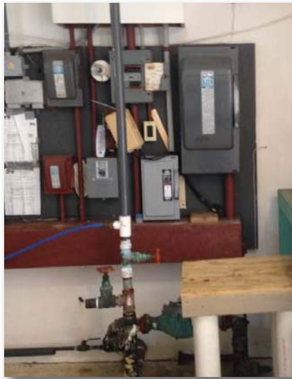
Water Pipe in front of Electrical Panel
