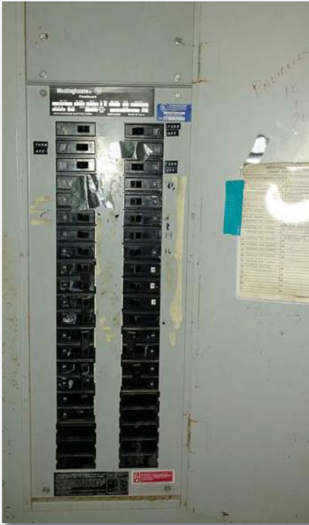
Electrical equipment well past typical 30 yr. life expectancy.
