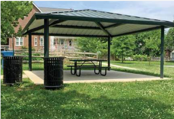
New ADA accessible Pavilion with new Trash Receptacles and seating.
