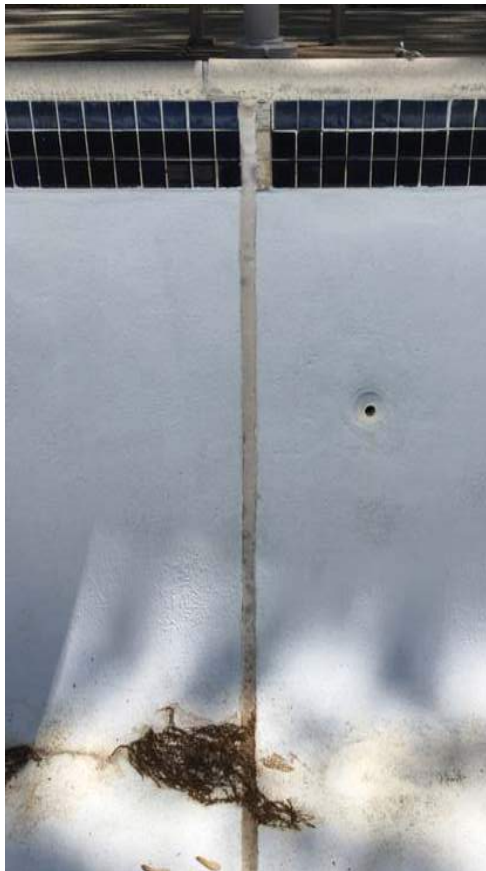
Coping Tile and Expansion Joint - Main Pool
